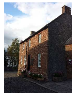
Robert Burns House, Dumfries
